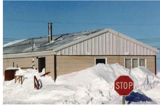
Snow banks insulate the ground, warming permafrost. Credit: RWDI Inc.
