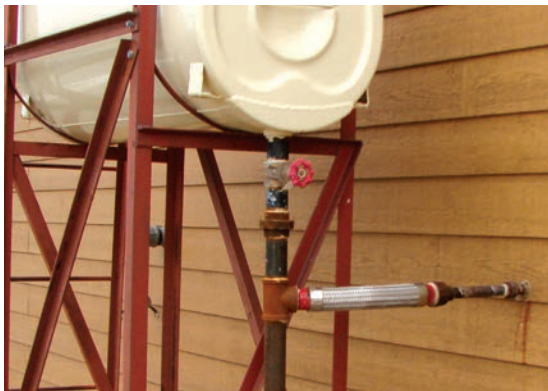
Flex hoses help prevent broken fuel lines.
