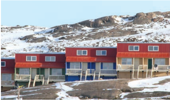
Owners of houses built on bedrock need to worry less about permafrost thaw.
