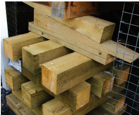
If you have a surface foundation, level your house as needed.
