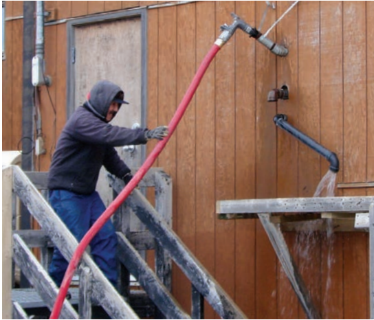
Overflow from your water tank can help thaw your permafrost.
