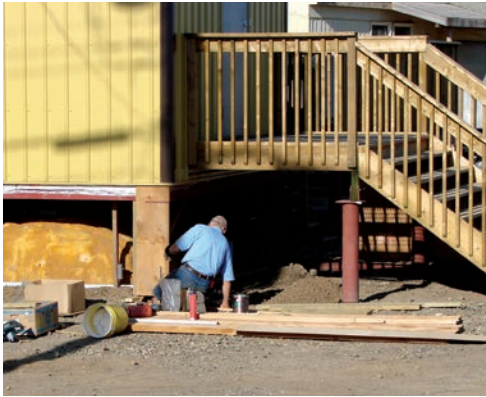
Proper maintenance of your foundation is important for your house.
