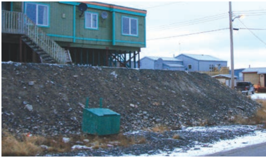
Thick gravel pads help preserve the permafrost.
