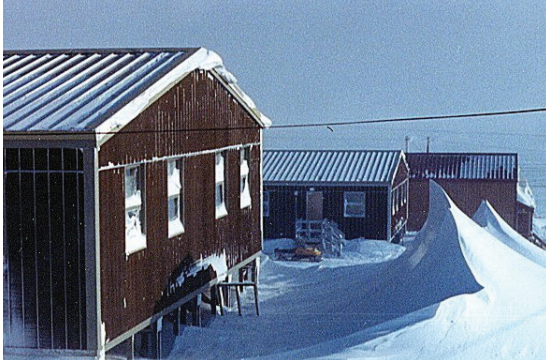
This snow drift is far enough from the house that it should not affect the permafrost. Credit: RWDI Inc
