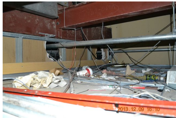
Left: The emergency lights are pointed in the wrong direction. Right: The holes in the fire separation wall are hazards.
