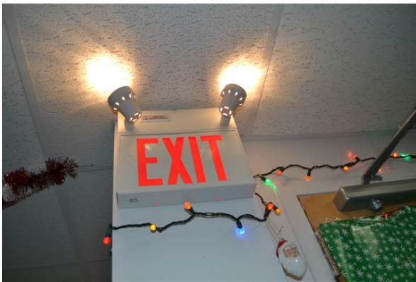
Left: The emergency lights are pointed in the wrong direction. Right: The holes in the fire separation wall are hazards.
