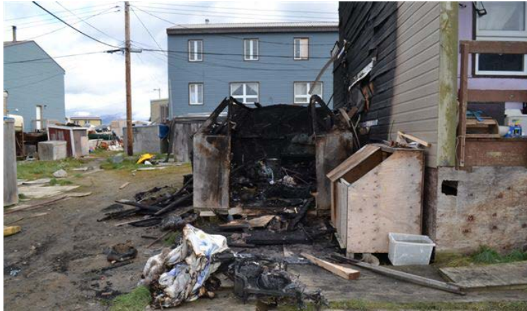
A shed and adjacent building are damaged due to fire. It should be noted that the shed is positioned very closely to the building.
