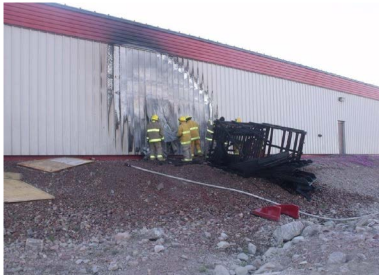
A fire in an empty crate damaged a commercial building. This could have been avoided with proper disposal of the crate.
