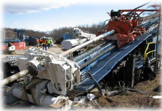
Figure 7 – Horizontal Drill Rig
