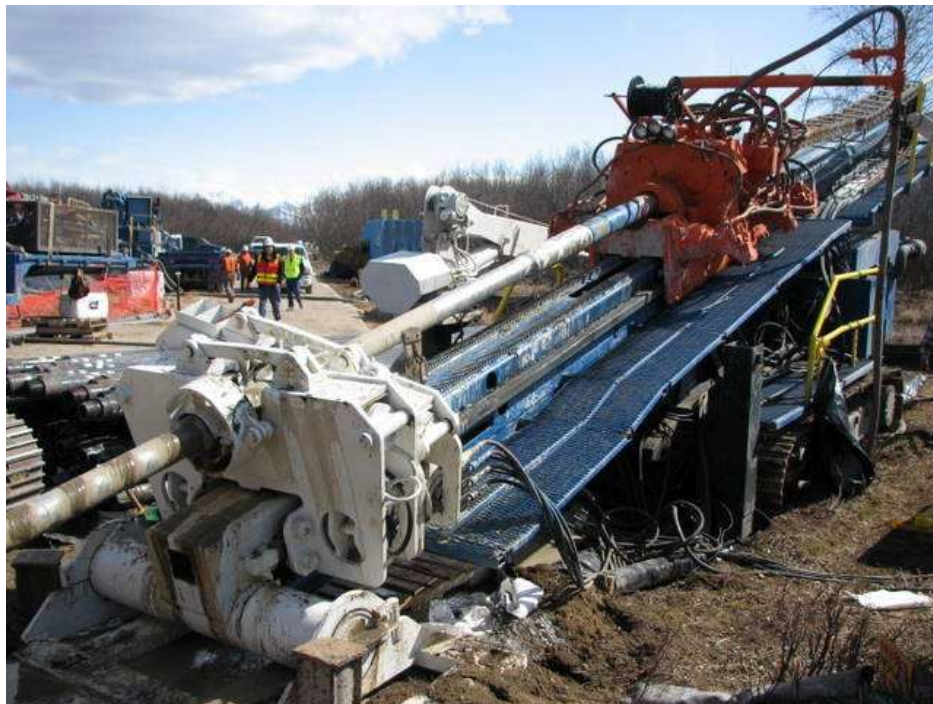
Photo: LTS – Horizontal Directional Drill for beach landing
