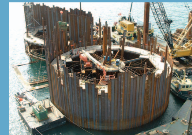
New Steel Sheet Pile Wharf Under Construction at Voisey's Bay
