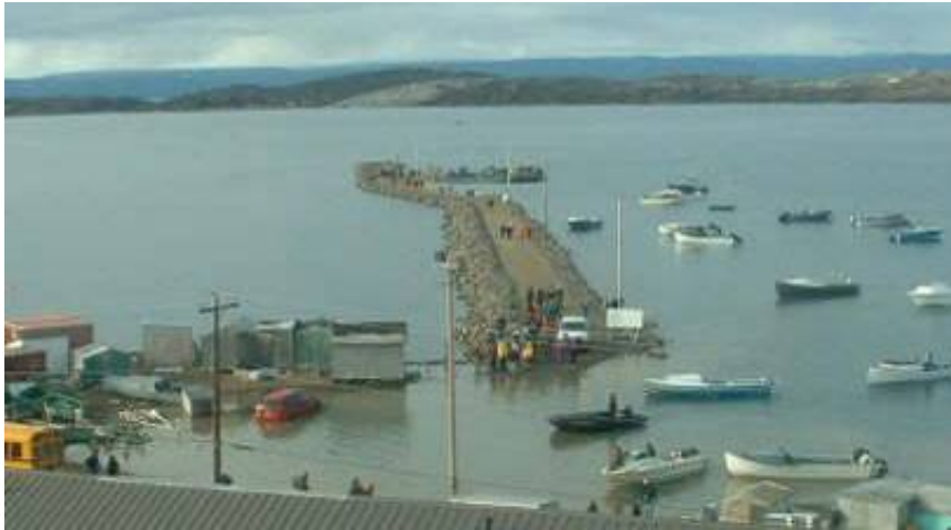
Figure N Municipal Breakwater during an extreme high water event, showing the approach and adjacent road flooded. The upper fixed dock can be seen at the end of the breakwater, with the lower fixed dock flooded.
