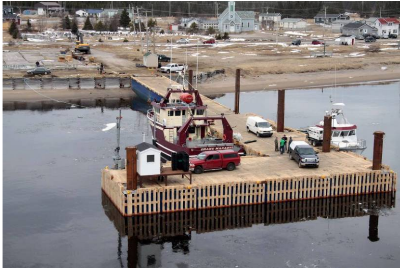
Figure V Small Craft Facility at Mingan, QC, showing a three-piece spudded float system that is completely removed during winter months. Photo courtesy Groupe Océan.
