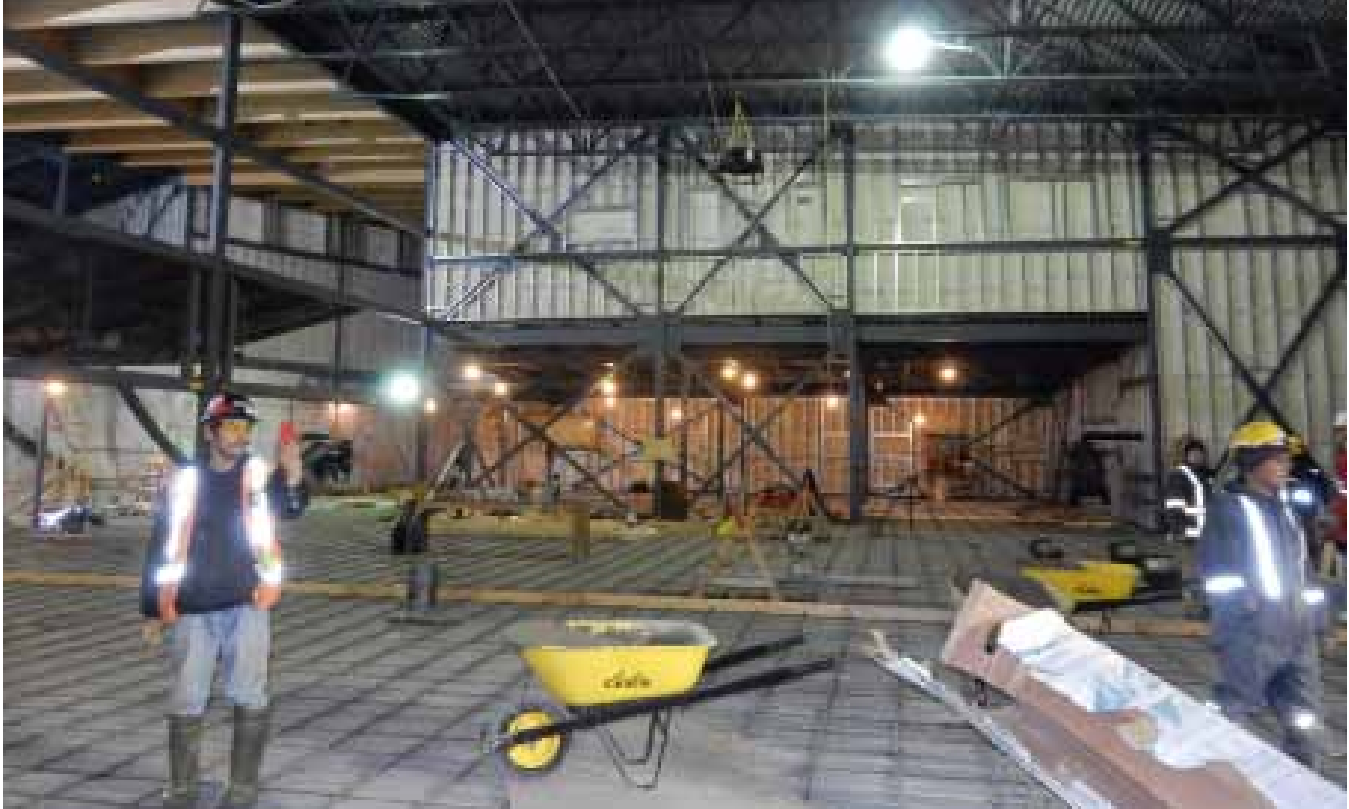
Construction of Tuugaalik High School in Naujaat.
