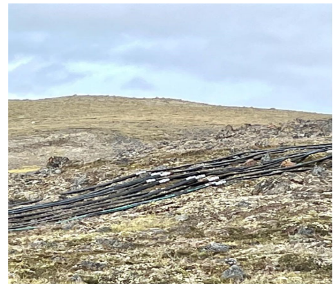
Figure 4: Picture of Supply Lines and Fittings installed on the land.
