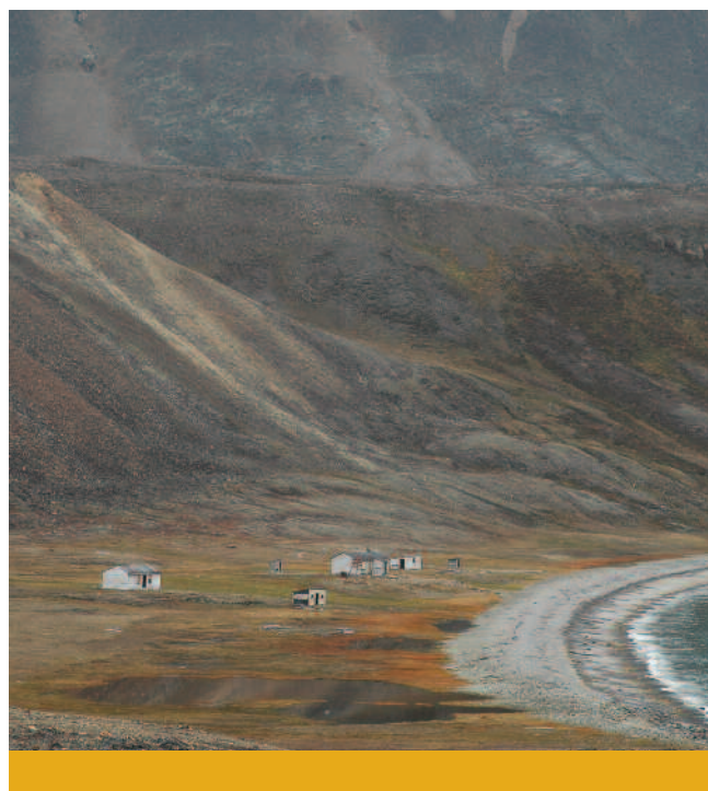
During Operation Lancaster in Aug. 2006, RCMP officers and Canadian Forces personnel participated in the grave restoration of two Mounties who died in the 1920s while stationed at Dundas Harbour on Devon Island. The buildings pictured here are what remain of the former RCMP detachment.
