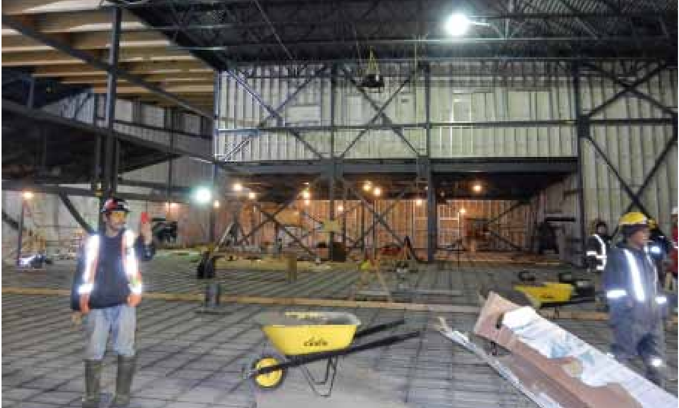
Construction of Tuugaalik High School in Naujaat.
